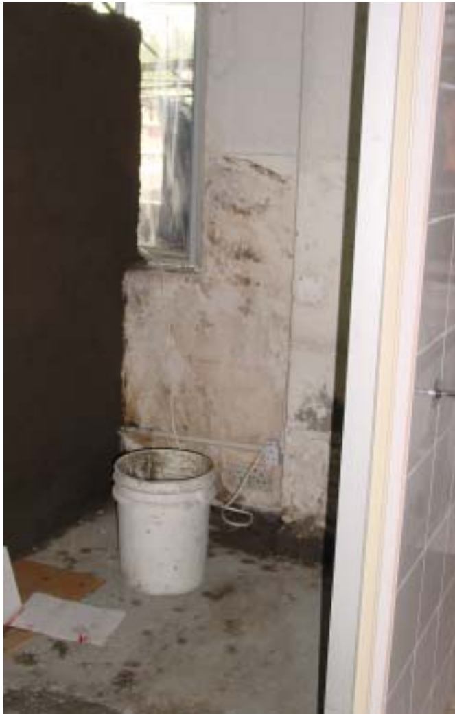
Picture7. The third toilet under construction
