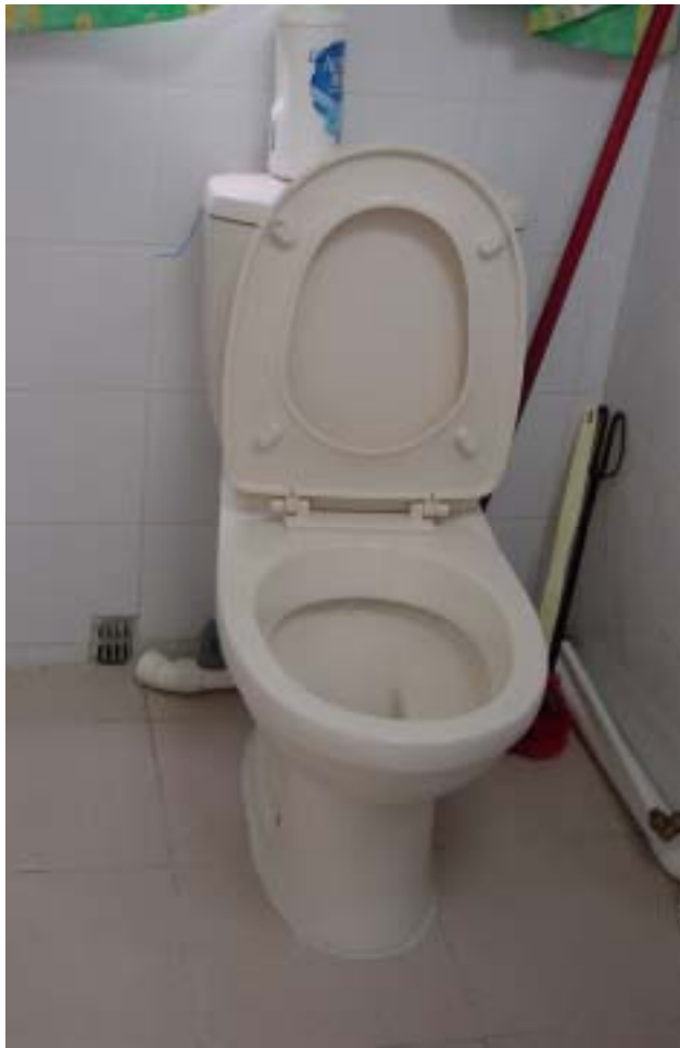
Picture 6. First new toilet installed in the afternoon of 4 September
